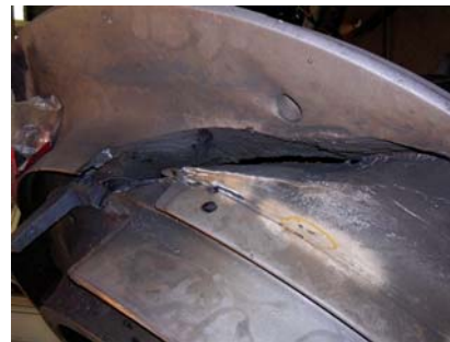
Detail of fatigue crack in the cone head
