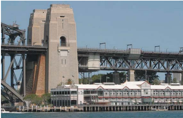
Sydney Harbour Bridge - repainting southern approach spans
