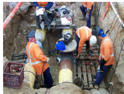
Preheating, temperature checking and monitoring on 500 mm nominal bore stopple tee
