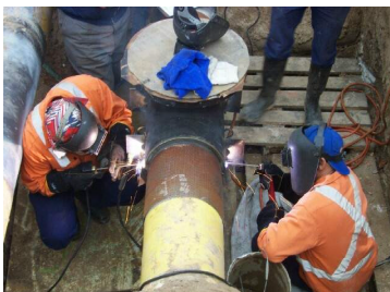
Welding of 350 mm nominal bore stopple tee
