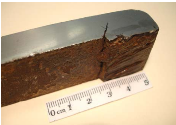
Figure 3. Typical furnace tube cracking
