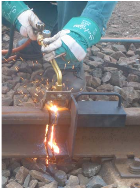
Figure 2. Cutting in progress showing wheeled nozzle guide running against cutting guide
